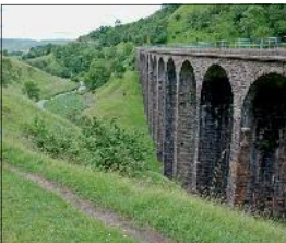
Smardale Gill Viaduct
